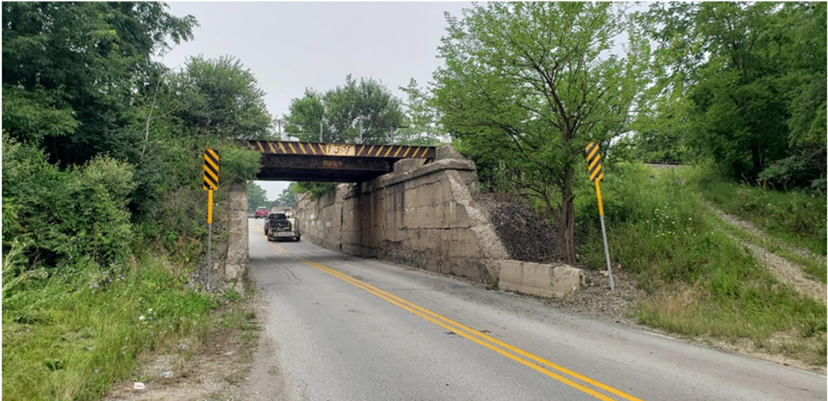
CSX/UP Railroad-Pauling Goodenow Road Underpass Structure
